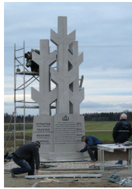
Construction of a monument at a location of historical significance
